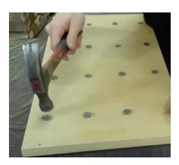
Place a split lock washer on each of (6) m5x18 machine screw place and a flat washer. Insert the screw into the pockets of the MDF bed section using the pocketed holes. Lightly tread a small t nut onto the screw. Repeat with the second bed piece. With both sections top down, place them side by side, lining up the pronged t nuts.
