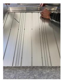
Install the second piece of angle near the middle. Once again, leave it loose so it can be slide back and forth.
